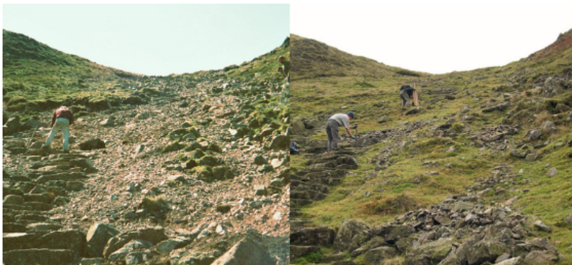
Fixing footpath erosion to conserve the area.
